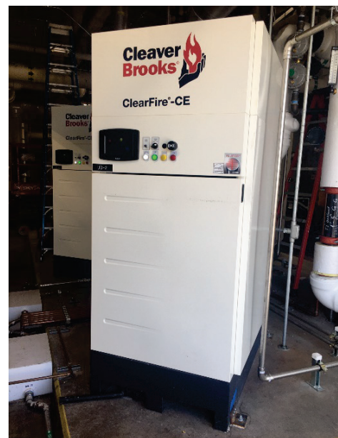
Figure 2 Example Condensing Natural Gas Boiler
