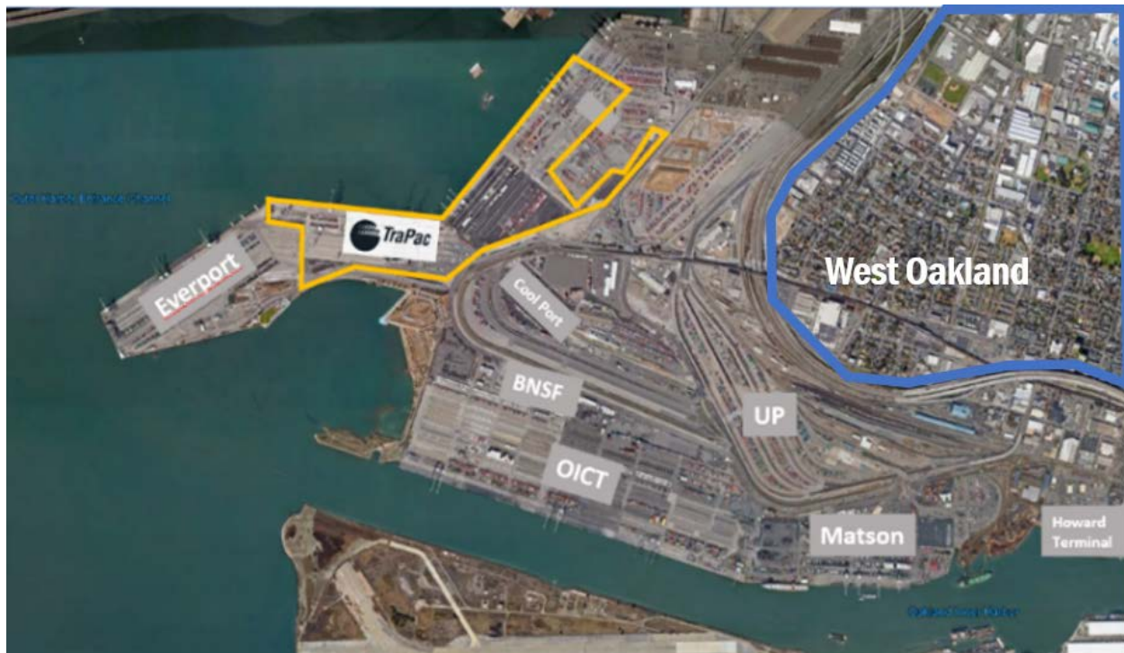
Figure 5 TraPac Terminal Area at the Port of Oakland and Proximity to the Historically Disadvantaged West Oakland Community
