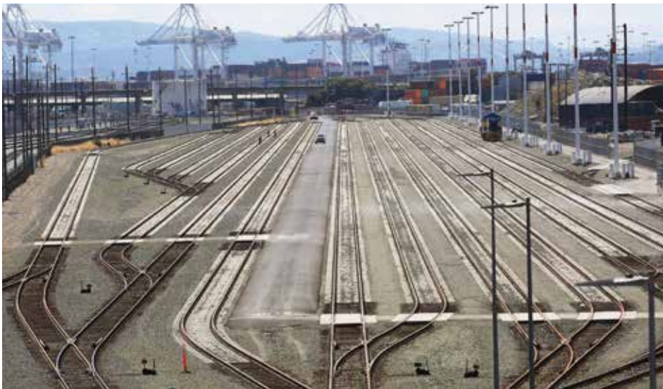
The newly constructed rail car storage terminal at the port of Oakland will allow rail shippers to deliver goods to the port. Credit Jim Wilson/The New York Times
