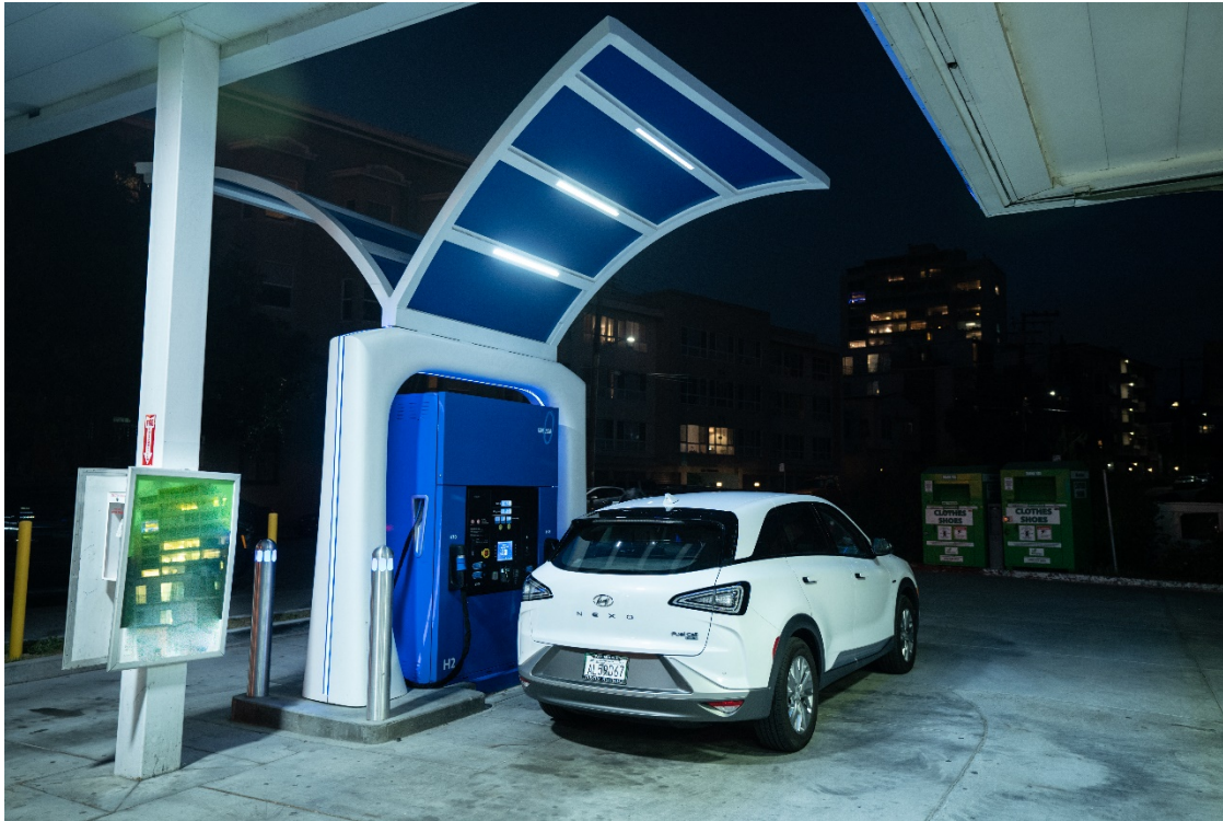
Figure 3 – True Zero Hydrogen Refueling Station
