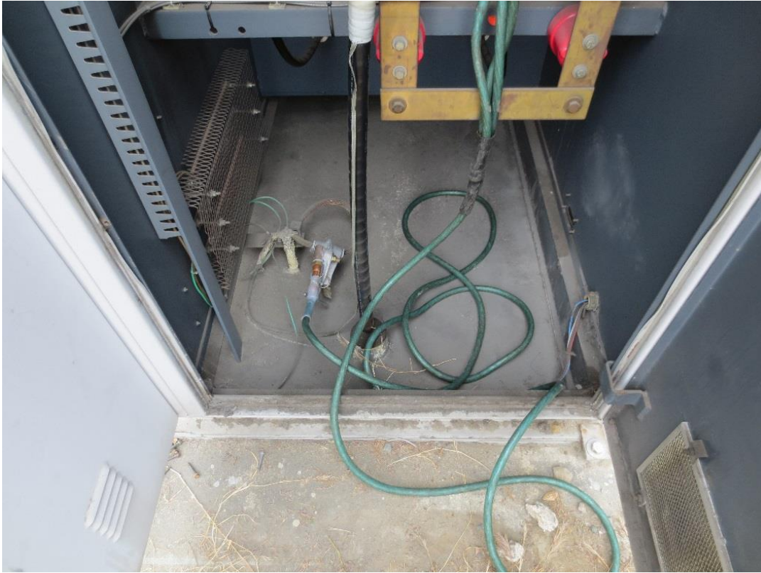
D. Existing Berth 24 Crane Switchgear Conduit Entry (Rear of Vertical Section 2)
