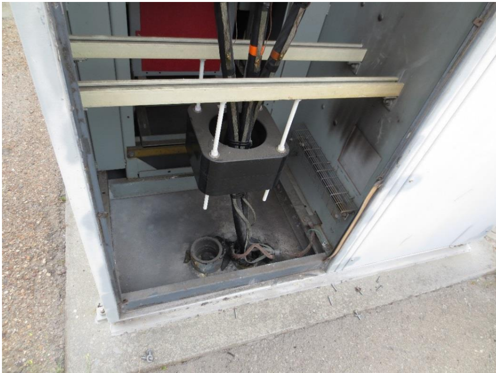
D. Existing Berth 23 Crane Switchgear Conduit Entry (Rear of Vertical Section 2)
