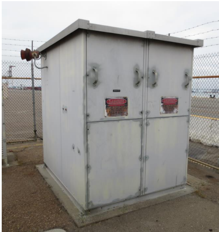
B. Existing Berth 23 Crane Switchgear (Rear)
