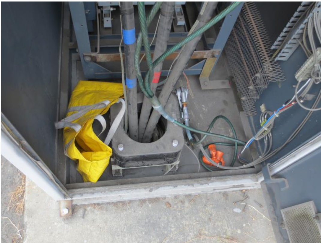
D. Existing Berth 24 Crane Switchgear Conduit Entry (Rear of Vertical Section 2)
