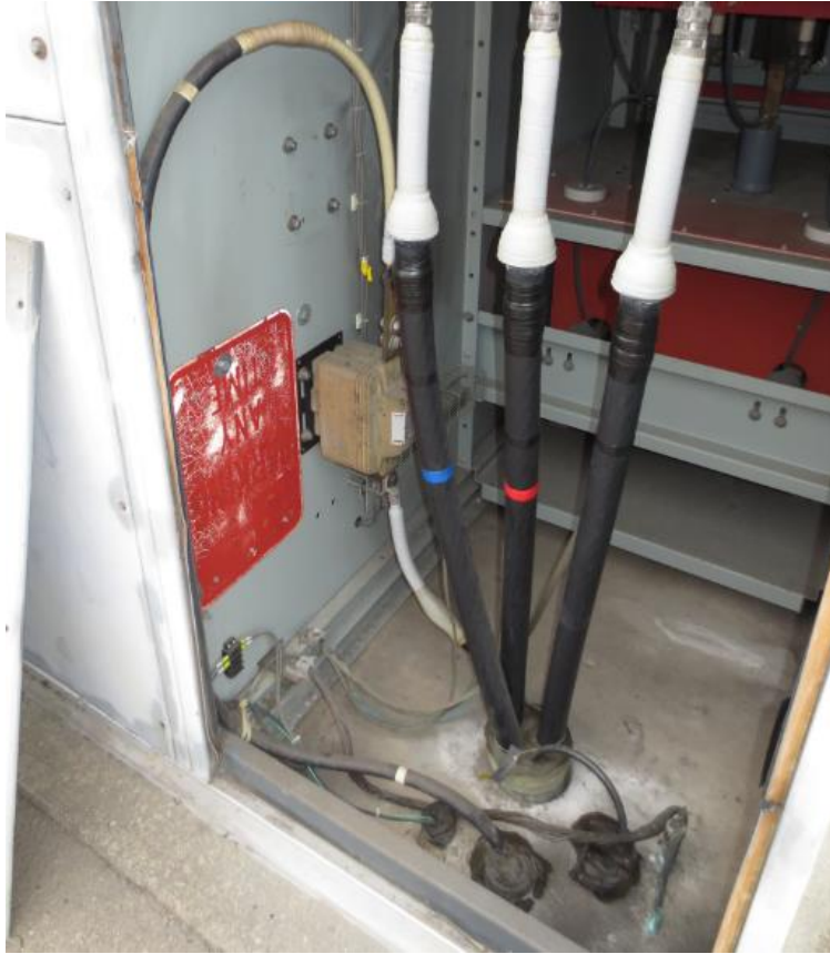
D. Existing Berth 23 Crane Switchgear Conduit Entry (Rear of Vertical Section 2)
