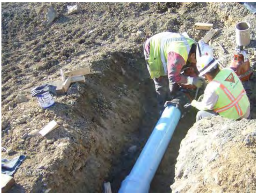
New water line construction
