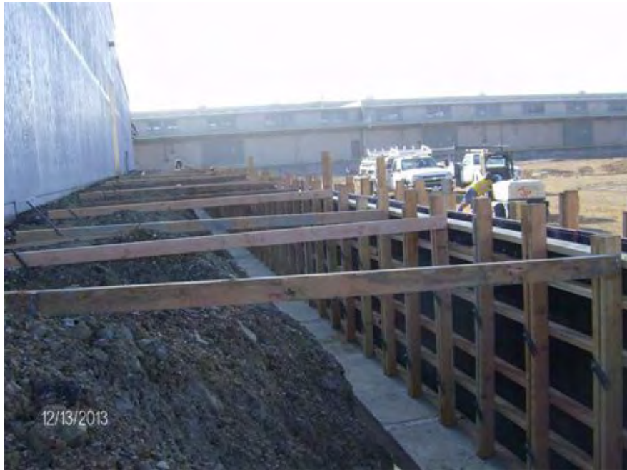
Framing for new retaining wall at new end wall
