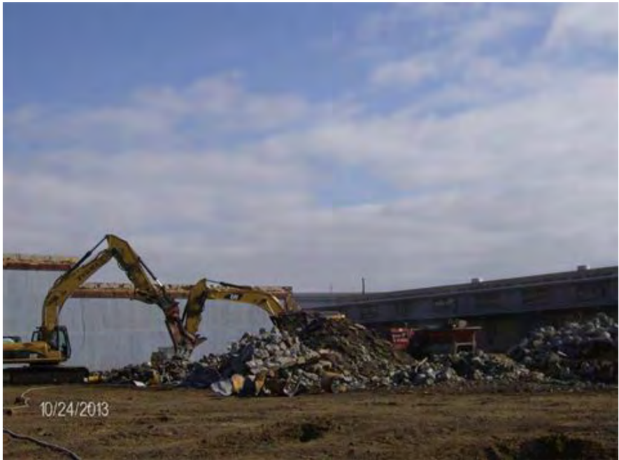
BBGB demolishing foundation of one of the middle bays
