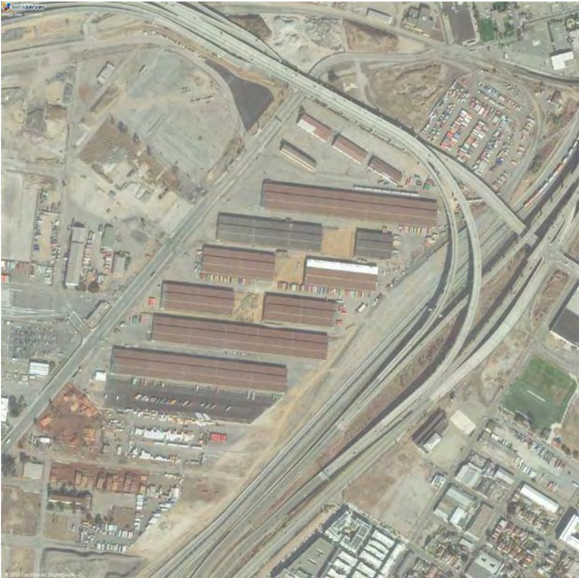
Nov 10, 2013 Aerial Photo Showing Rail & Warehouse Demolition Work
