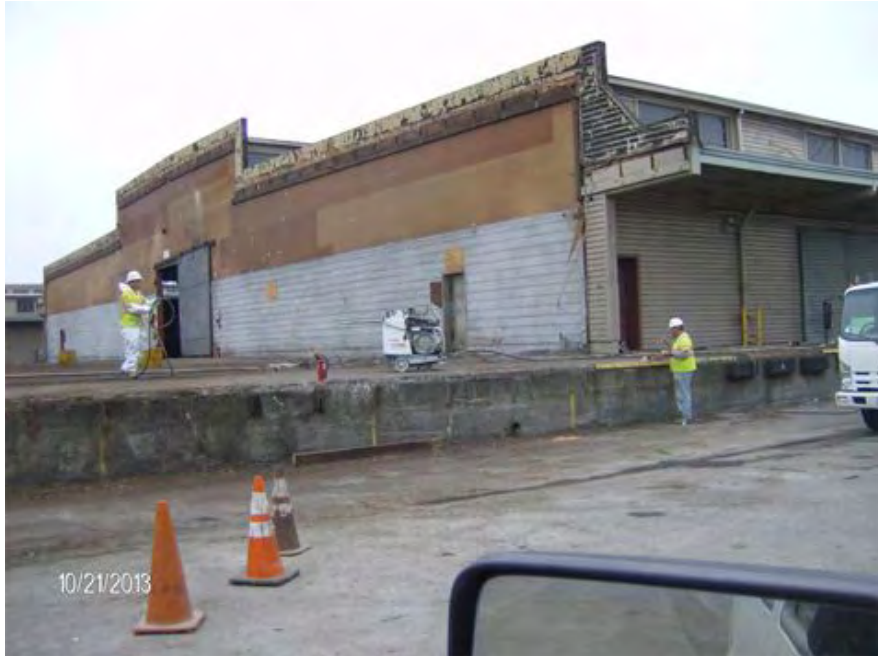
Beliveau installing exterior siding to new end wall on deconstructed building
