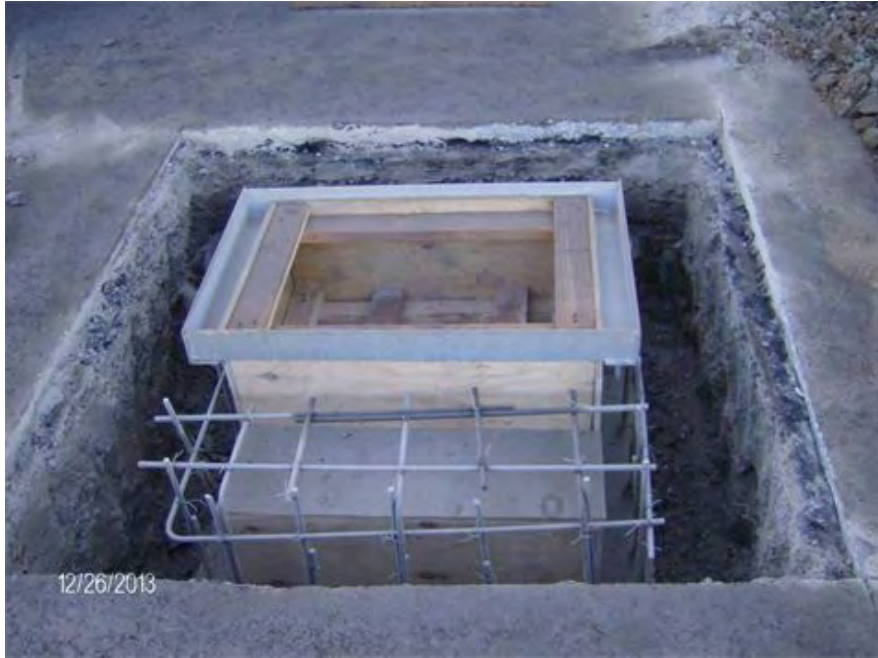
Installing new storm drain catch basin
