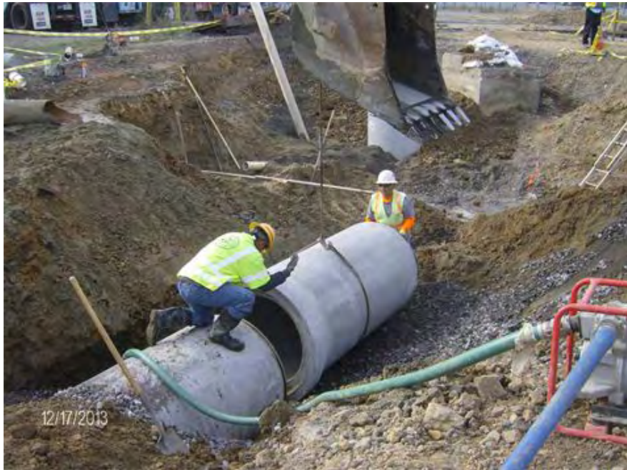
BBGB installing new Storm Drain connection to Maritime Street
