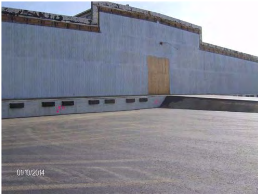
Finished pavement at warehouse preservation site
