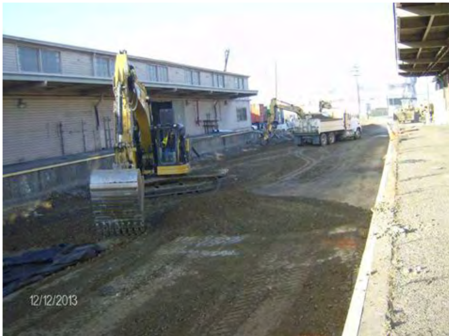
BBGB constructing new access through 18 th Street
