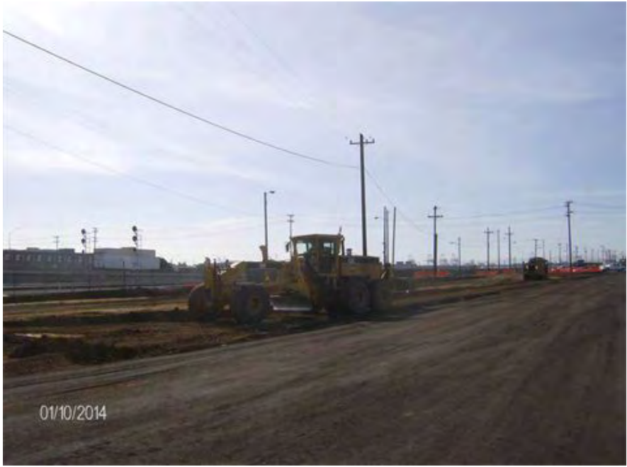
Grading sub-base for New Rail Yard
