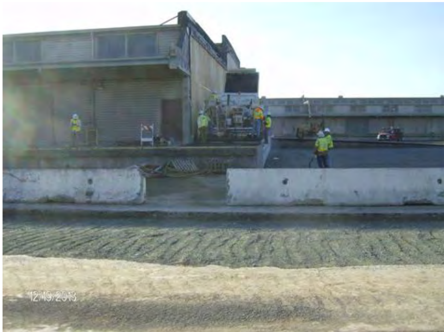
Paving at warehouse preservation site
