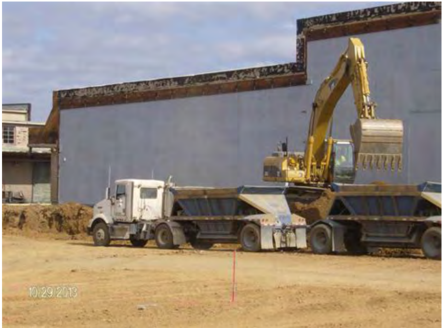
BBGB removing soil supporting the raised slab of middle bay
