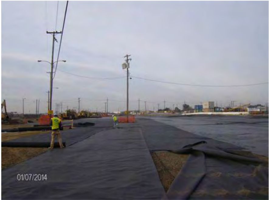
Placing geotextile fabric to strengthen sub-grade soils
