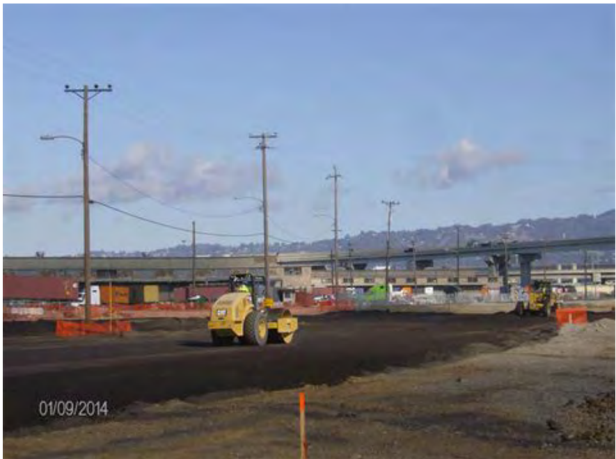
Placing Aggregate Base for New Rail Yard
