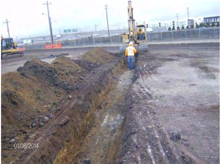
Excavation for rail yard storm drain system
