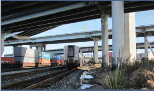
Figure 7: I-80/I-580/I-880 Interchange Looking North
