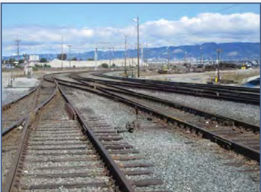
Figures 4, 5, & 6: 7th Street Yard Lead Tracks
