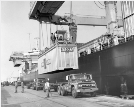
Shipboard cranes on the Elizabethport, Sea-Land Terminal, Oakland, September 17, 1962.
