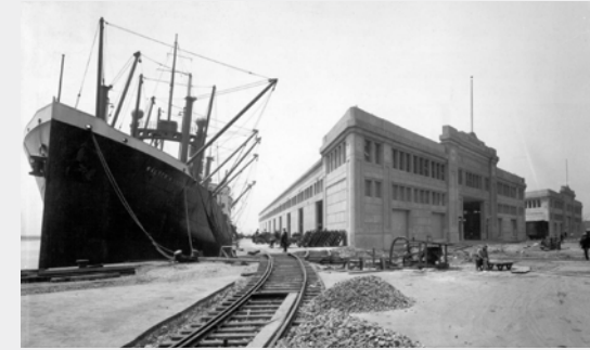
The Port of Oakland's Grove Street Pier opened in 1928 between Grove and Jefferson Streets, on the site of Municipal Dock No.1.
