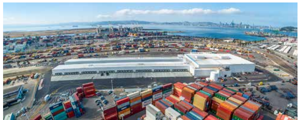
Cool Port Oakland - refrigerated distribution center
