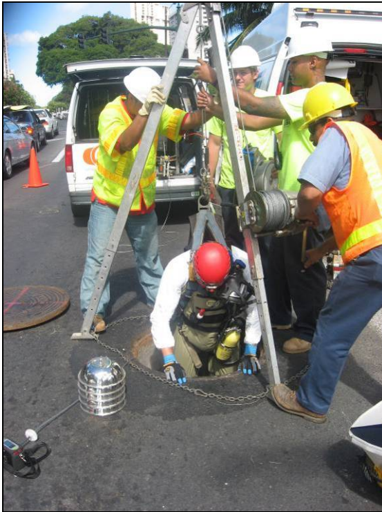
Photo 1. Confined Space Entry
